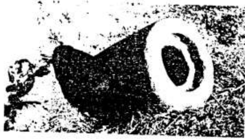
5. Ephesos block from stone pressure pipe, showing recessed male-female joint. Also to be noted are the two small holes, one on top and one in the side of the block; their purpose is uncertain
